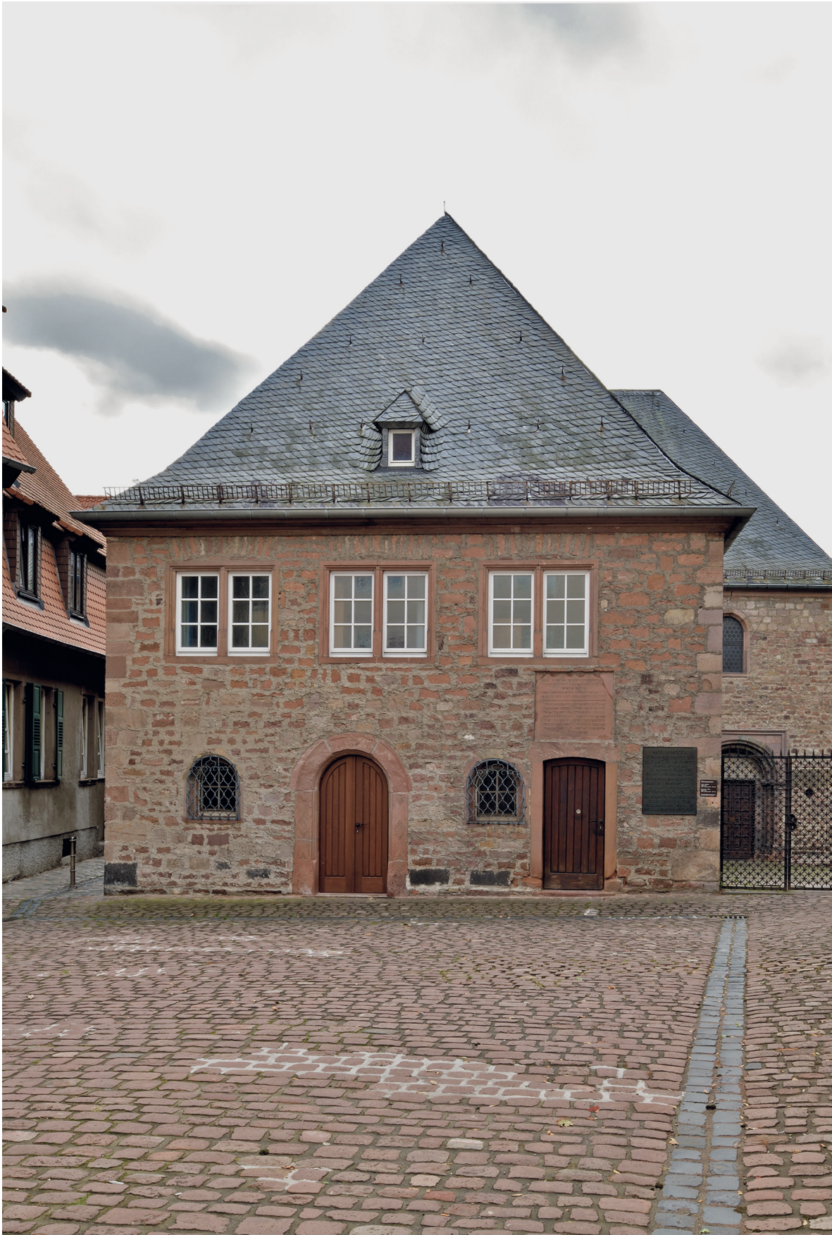
Fig. 408: North façade of the Jewish council chamber and the entrance hall to the women's shul in Worms Synagogue Compound, current state
