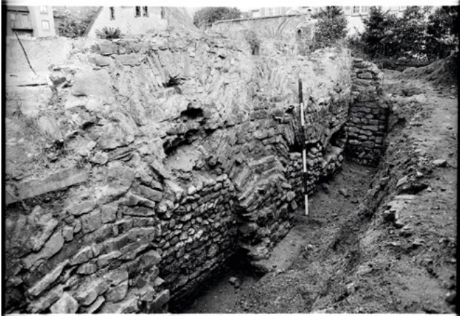
Fig. 32: Excavation of the medieval cellars of the former community hall before the building of today's Rashi House . Historical photograph, 1980
