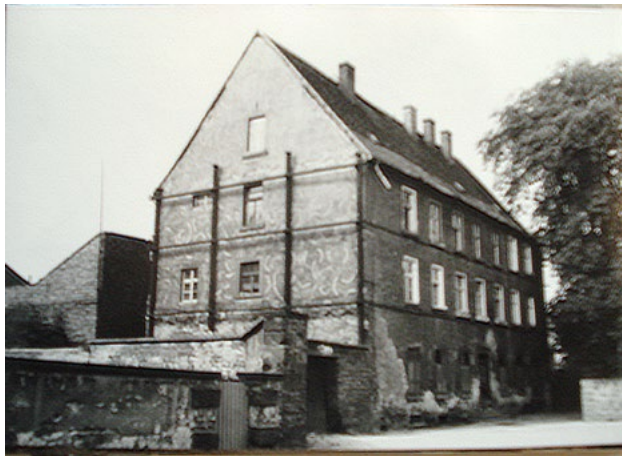
Fig. 29: The former Old People's Home of the Jewish Community Worms, in dilapidated state. Historical photograph, c.1968-1971
