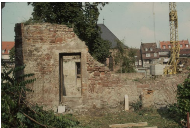
Fig. 39: Preserved rising masonry of the west wall of the former community hall, 1980
