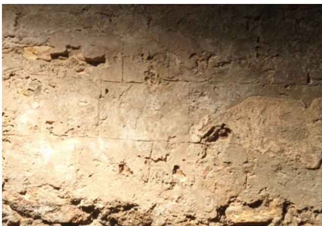
Fig. 42: Romanesque plaster areas with characteristic pietra-rasa rendering in the medieval cellars of the Rashi House , 2020
