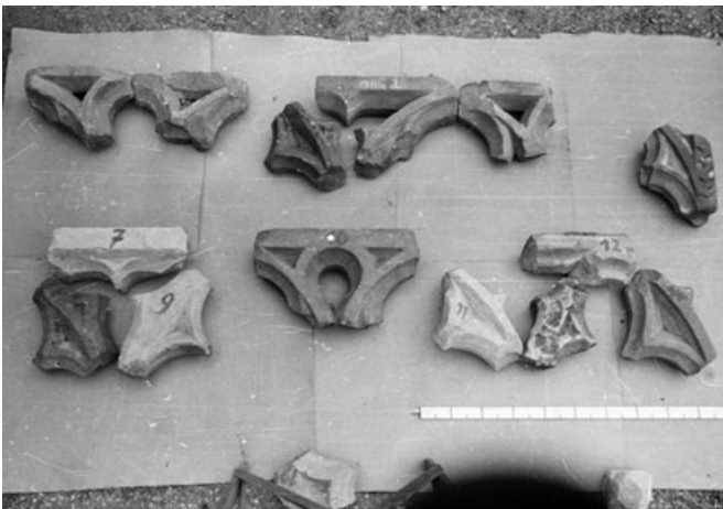
5. Example of the systematic sorting of the original fragments. Historical photograph, after 1945
